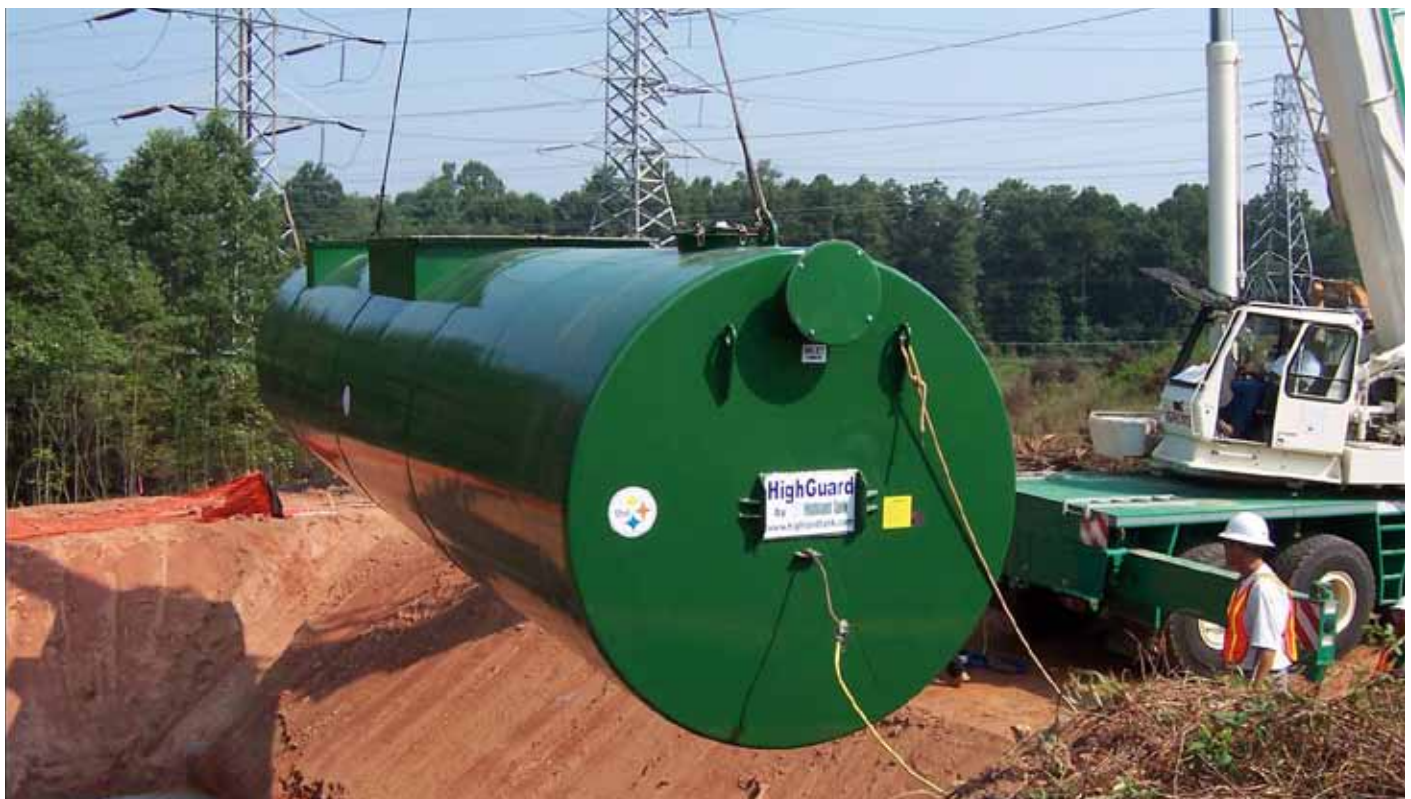
Belowground oil/water separators are usually of double-walled construction with electronic leak detection.
