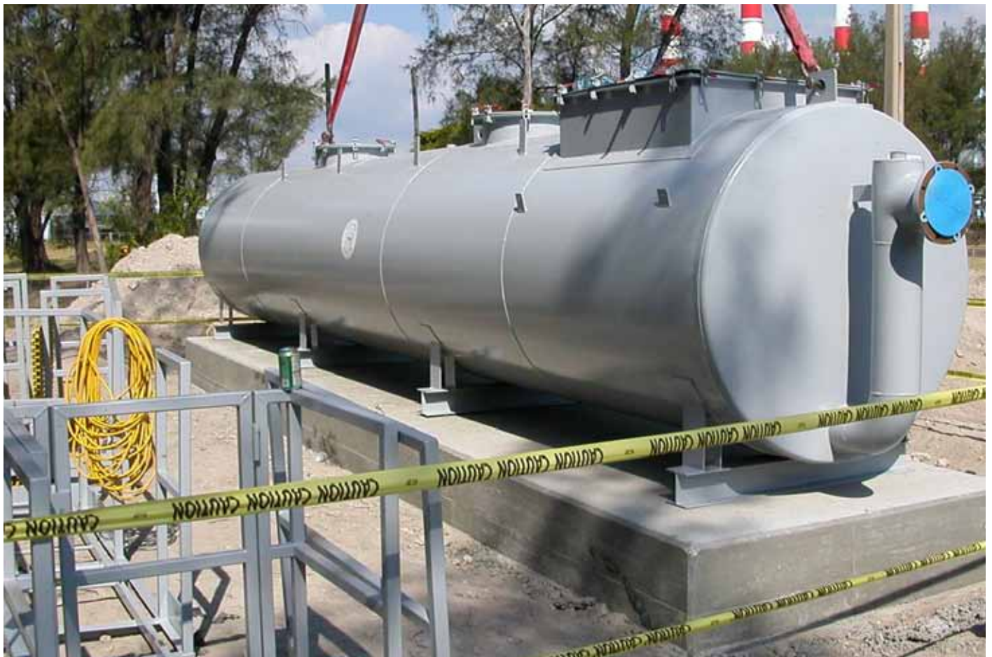
Aboveground oil/water separators are supplied with pre-engineered collection basins with non-emulsifying influent pumps and controls.
